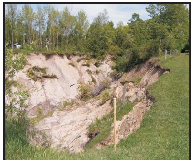
Gully at Bluewater Beach, June 2010.
